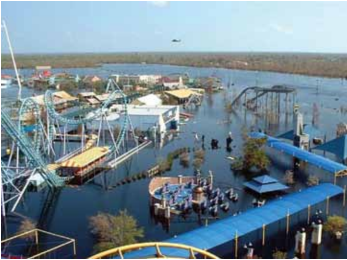
Six Flags New Orleans under water after Katrina.
