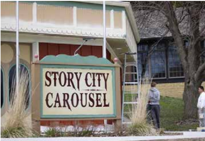
The Story City carousel building renovation continues.
