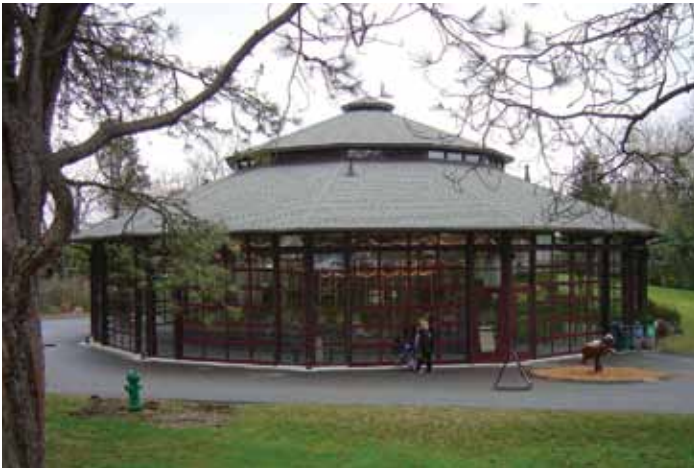
Another impressive Polygon carousel pavilion is at the Woodland Park Zoo in Seattle, WA. The glass curtain walls are easily opened up on warm, sunny days, or closed tight to protect the historic 1918 PTC #45 carousel inside.
