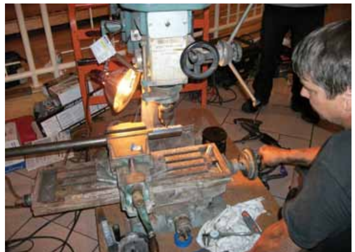
Key-way slots being milled on site at the mall.
