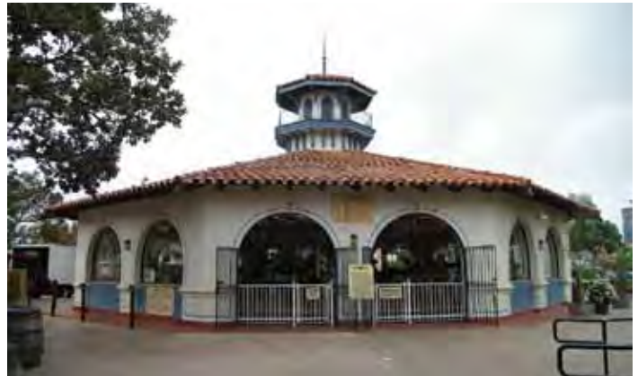
The Seaport Village Carousel Building now houses a 1905 Looff with a mix of Looff and Carmel figures dating before and after the construction of the mechanism.
