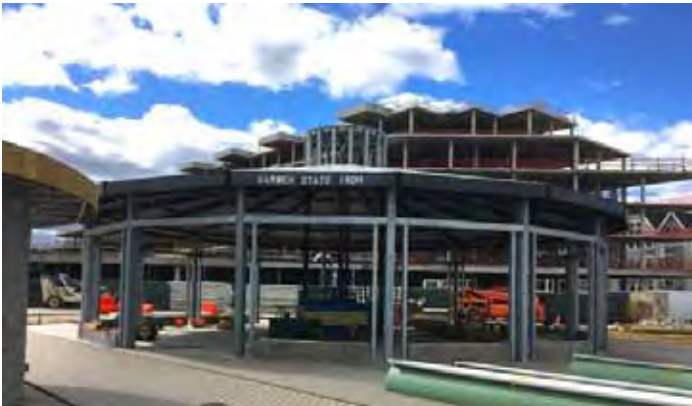
Carousel building for new carousel in Long Branch, NJ.
