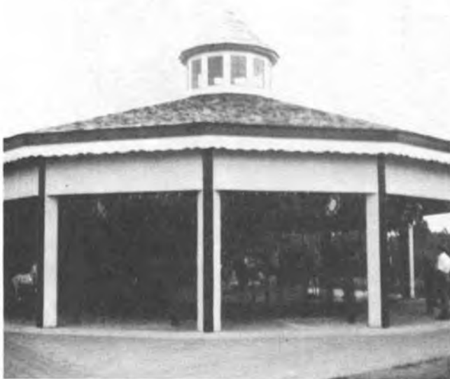
A new carousel building
