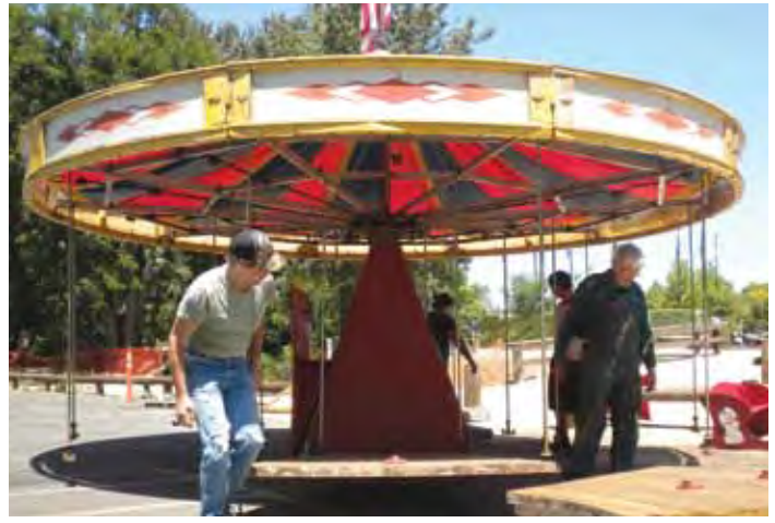
The basic tower set up with top on and one floor panel.
