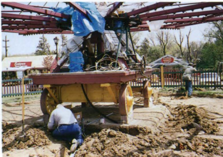
Preparing the site for the carousel included extensive construction and landscaping.
