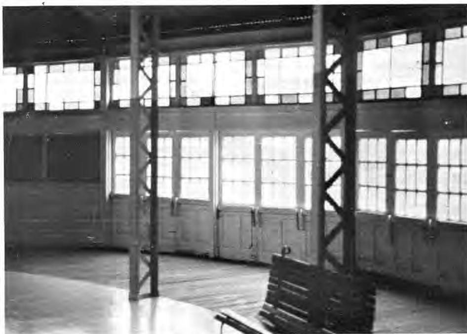
This photo shows the outer, inner and roof steel supports, and lower row of windows and doors. The beautiful stained glass windows are made of Sandwich glass and can't be found or reproduced today.
