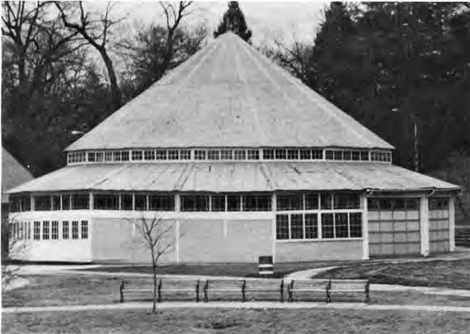
The carousel building in Roger Williams Park is possibly the first prototype of its kind in New England and possibly the only structural steel framed and corrugated iron roof Victorian carousel structure left anywhere today.
