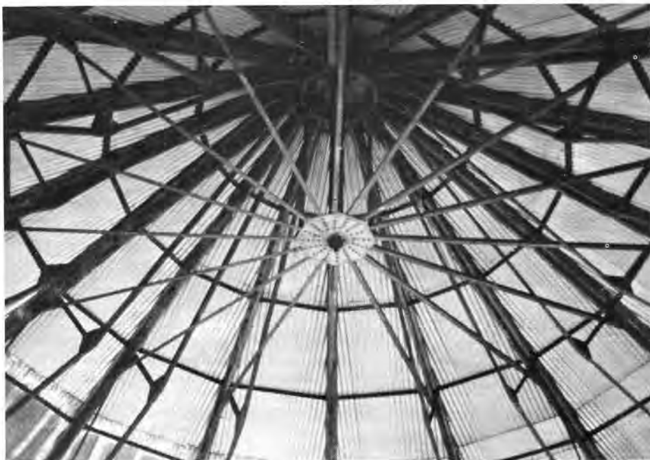
The peak of the building from the inside with its structural steel configuration. This building is slated to be replaced with a new Victorian-style building just across the street.
