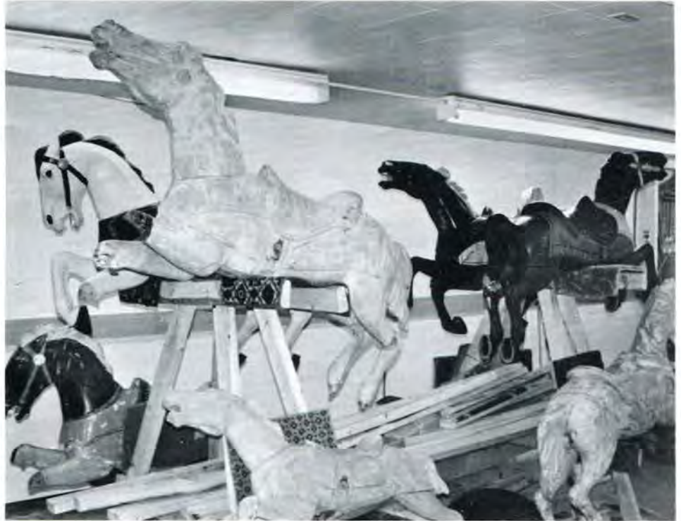
About two months after the Teton Dam flood carried away at least four of the horses and inside movable panels on the Rexburg Spillman Carousel, vandals used a sledge hammer and ax to hack off feet and legs from the horses.
