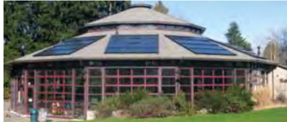
The customized Poligon building at the Woodland Park Zoo in Seattle, host to PTC #45, has added solar panels. Photo courtesy of www.jeasolar.com
