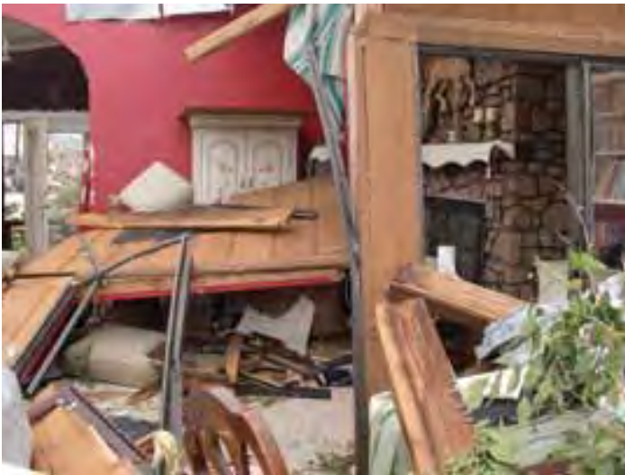
Only a small portion of the living space around the fireplace was left standing after the tornado.
