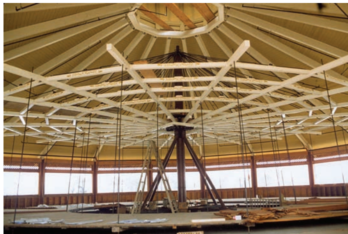
The mechanism during installation at Shoreline Village in Long Beach, CA, in 1983. Barbara Williams photo.
