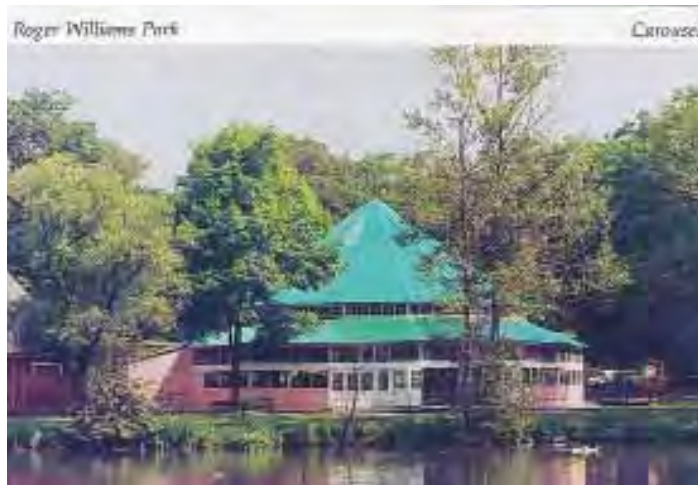
The old carousel pavilion, built around 1895, at Roger Williams Park, near the Dalrymple Boathouse.
