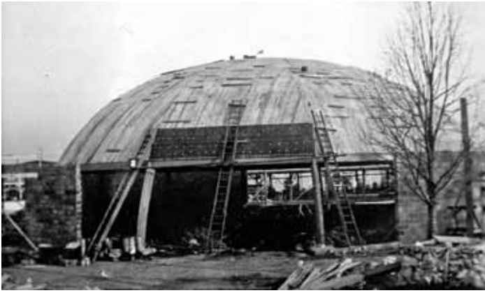
The new carousel building under construction in 1944-'45. Photo courtesy of John and Margaret Winkler
