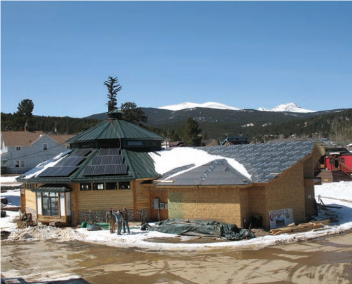
The carousel building, shown here in mid-March, should be nearly complete by the time you read this.
