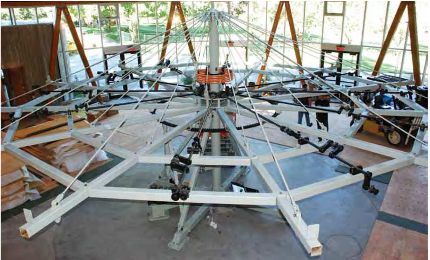
The carousel frame takes shape at Butchart Gardens during installation. “This carousel will be around long after you and I are gone. Though I was not there for installation, I did help load every inch of that steel into the semi. No doubt that a century from now, children will be enjoying rides on The Butchart Gardens Rose Carousel.” – Roland Hopkins.
