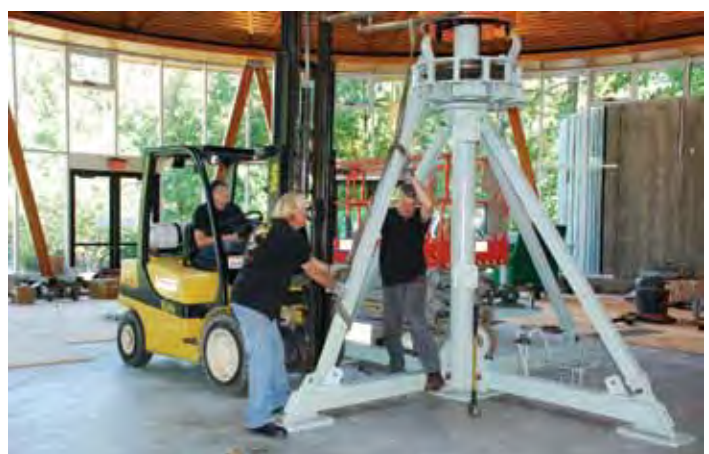
The rest of the supports for the center pole go up.
