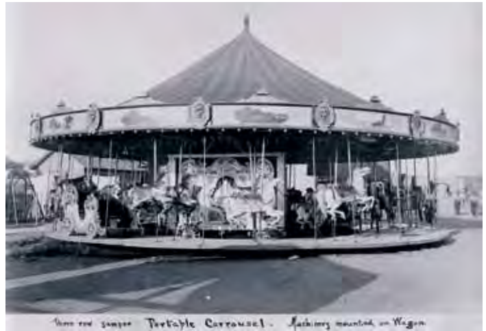
Three row jumper Portable Carrousel. Machinery mounted on Wagon
