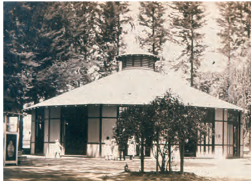
The original carousel building in Urbita Springs, CA, was designed by Oliver Davis as a modular structure and would eventually move with the carousel to San Diego.
