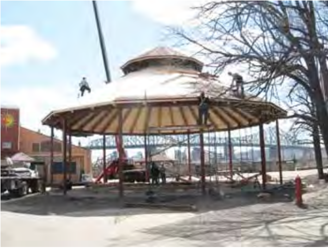
The new carousel building goes up at LaRonde.
