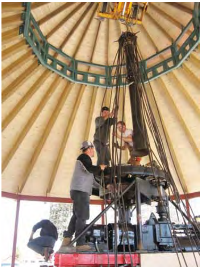
Raising the center pole.
