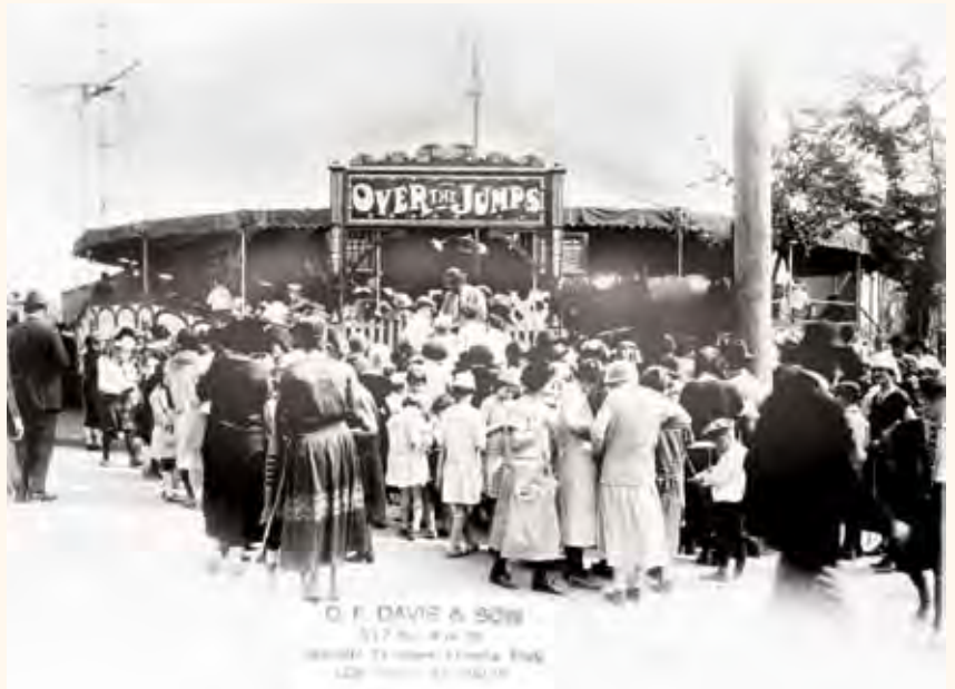
Spillman Engineering "Over-the-Jumps." Lincoln Park, Los Angeles, CA. Date unknown.
